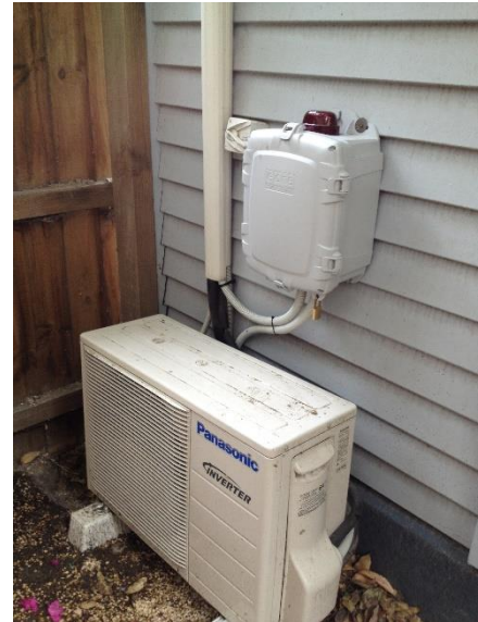
(Typical Alarm Panel Instalation)
